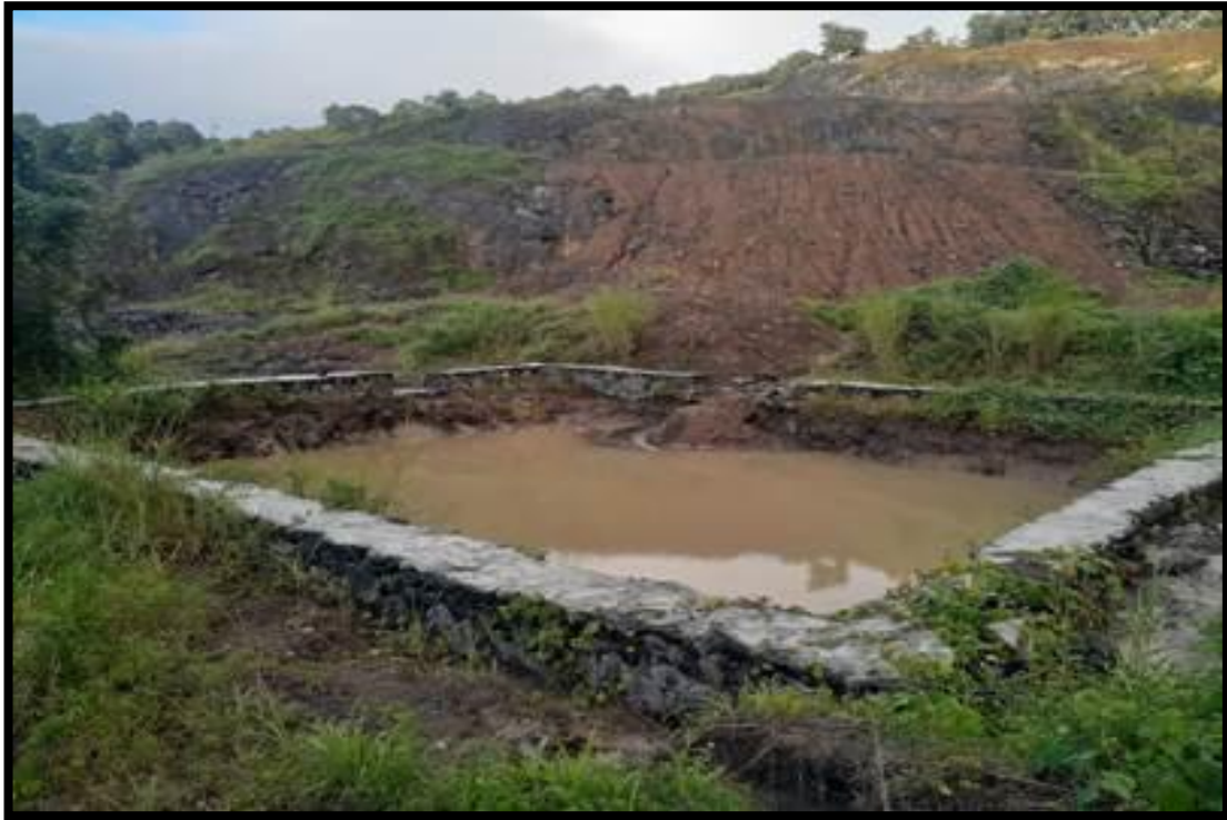
Rain Water Collection pond
