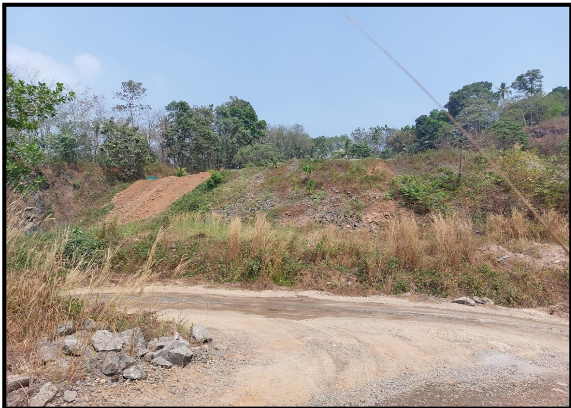
Over burden stacked in designated place within project site
